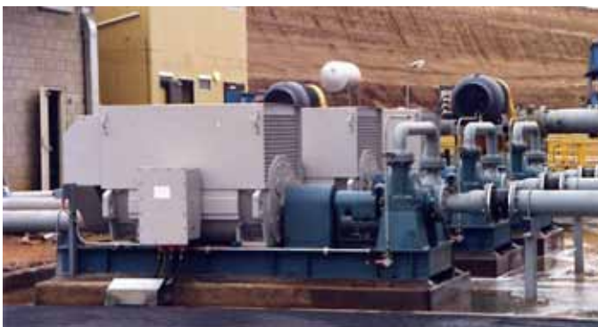
Gold Tailings Pumps in Australia - 3700 4x6-19
