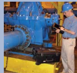
Technician installing wireless, internet-enabled RESolve instrumentation.
